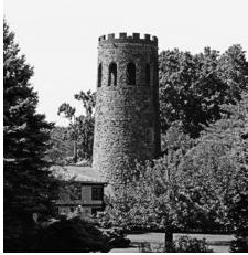
Located at the northwest edge of the estate, this large fieldstone water tower remains as one of its most distinctive outbuildings. It was originally taller, and had a conical roof with a windmill on top and a water wheel. Some brackets are still visible on the highest section. The roof was originally supported by posts located on the interior of the structure, which also held a narrow walkway.
