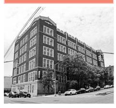
Designed in the Collegiate Gothic style, this prominent five-story structure was built of solid brick exterior walls with limestone and decorative terra cotta details. Its floor and roof are concrete slabs supported on concrete encased steel beams that are, in turn, framed into the masonry.
