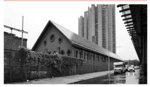
Situated along the west side of Jerome Avenue just south of Mosholu Parkway, the High Pumping Station is a long and narrow red brick Romanesque Revival building topped by a steeply pitched roof. The façade is divided into a series of bays, each consisting of two arched windows flanked by shallow brick buttresses.
