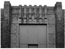
Substations convert high voltage alternating current (AC) to low voltage direct current (DC), used to provide traction power for the trains. In the early 1930s, manually operated substations became obsolete, which impacted the design of the structures that housed them. Most of them were replaced by smaller underground vaults, and those aboveground were constructed in a simple Art Deco style.
