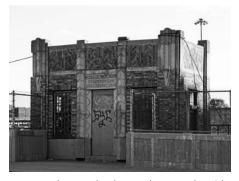
Located along the south side of West 205th Street, these structures were built next to one another to form a gateway to the yard, and are connected by an iron bridge. Each building is actually three stories tall, but only the top story is visible from the street. The façade of each one is divided into three vertical segments by limestone columns, connected by a wide limestone cap along the roof line. Above each of the three bays, the brick is set in a striped herringbone pattern.
